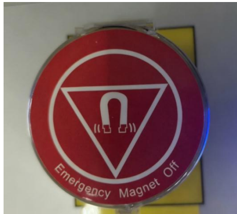
Fig3 Warning: Emergency Magnet Off
